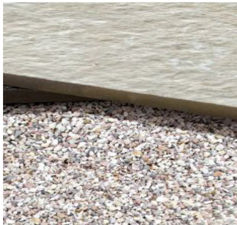
LAYING OVER SAND
