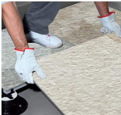
INSTALLED AS A FLOATING FLOOR
