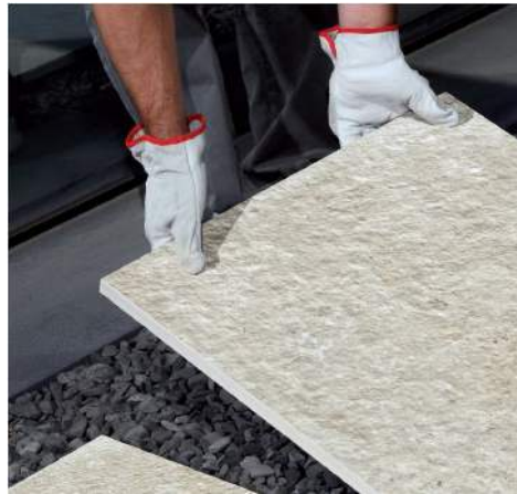
LAYING OVER GRAVEL
